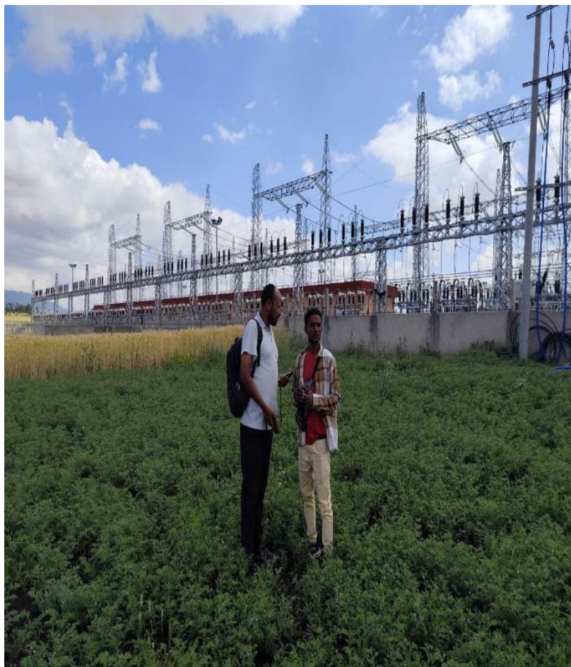
Figure 6 Survey work for UG line crossing farmland authorities located along Koye Substation (before harvest)
